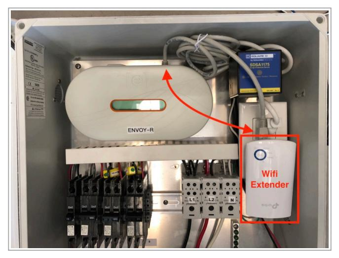
NOTE: It may be necessary to restart the energy monitor so that it can be associated with the new extended WiFi network.
